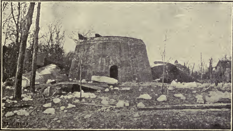
FIG. 6.—GENERAL VIEW OF RUINS OF THE ELGIN STAND-PIPE. ( Eng. News. )
